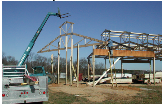
Work in progress, with the two man crew from Koenecke installing trusses. The building went up very quickly, with not a wasted moment!
