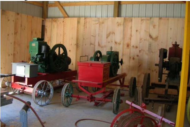
July 14 Partial installation of paneling in the F&J annex. Lyle Opperman and Jim McGhee planed the lumber, cut it and installed it. A trim board or molding is planned for the top.
